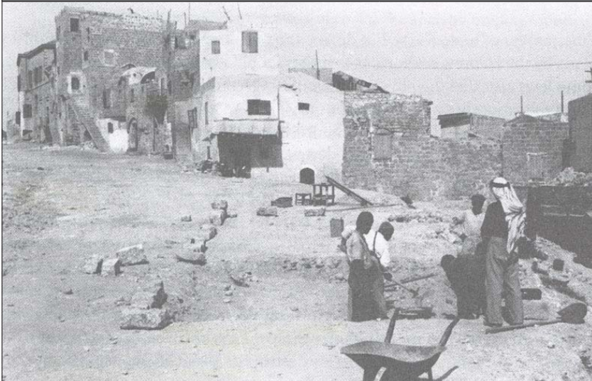
Photo 4.2: Excavating Destroyed Jaffa Neighbourhood
